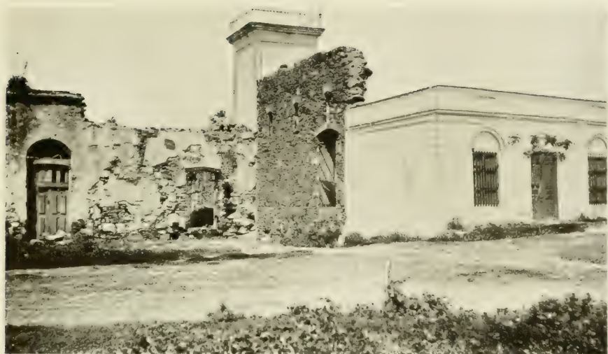
COLONIA : RUINED FORTRESS WALL.
